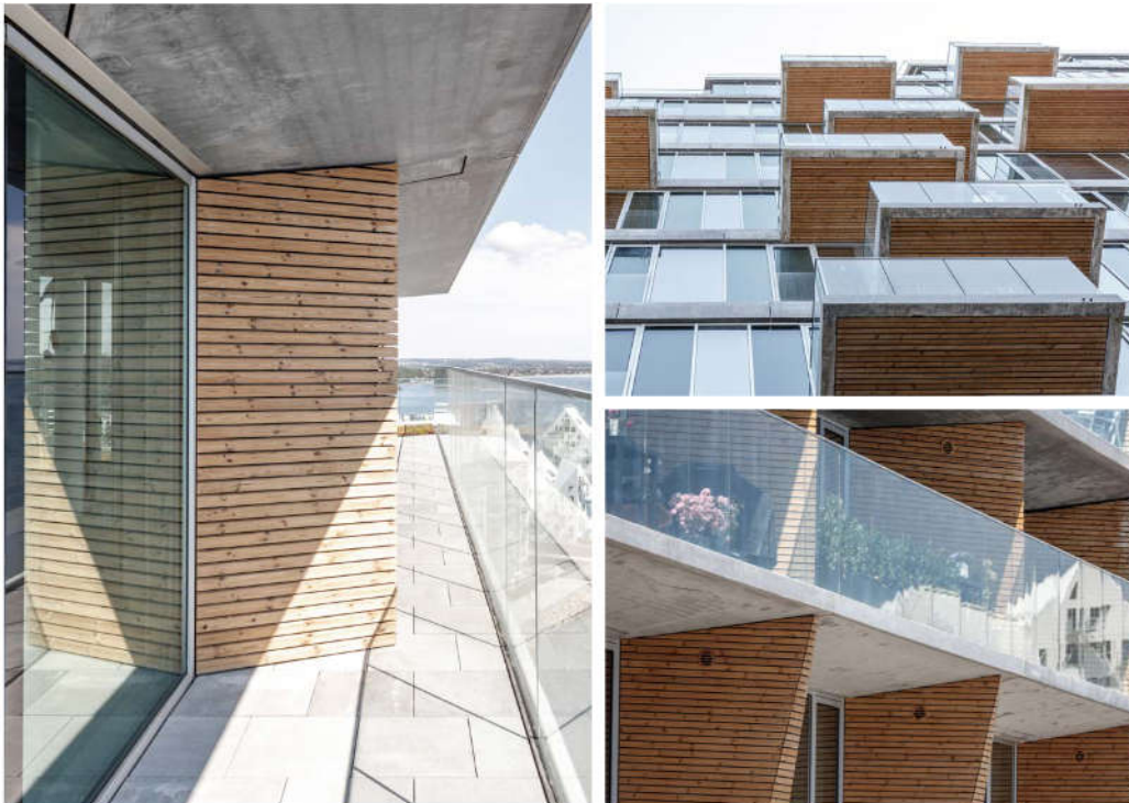
Thermo pine / Apartments / Bjarke Ingels group- Aarhus - Dolle nordic a/s / Denmark / © photography Dolle.
